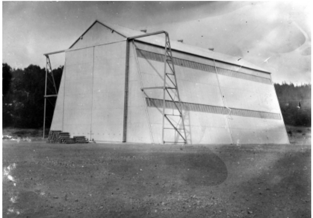
Ft. Scott Balloon Hangar, San Francisco, circa 1939 (now demolished). (PARC, GOGA 32422)
