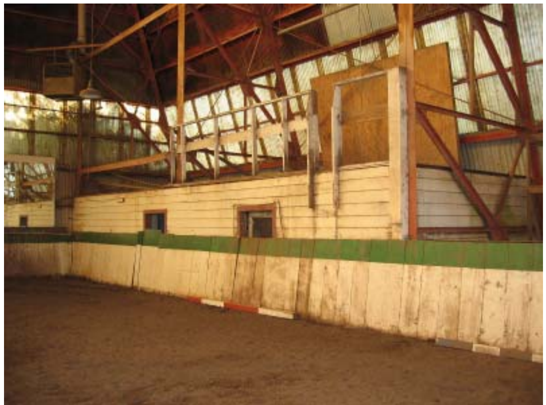
The southwest interior corner of the Balloon Hangar shows the original vertical trusses, rooms built during the Nike Assembly use of the building, plus the wall of the current indoor riding rink. (John Martini, 2003)
