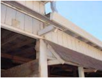
Motor Vehicle Shed interior showing 4x4 post and beam and cross bracing. (John Martini, 2004)
